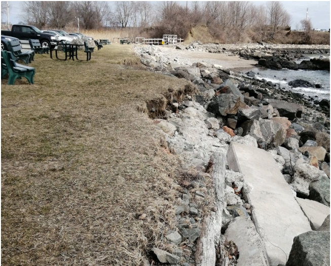
Erosion of the coastal bank from storm surge and increased sea level associated with climate change
